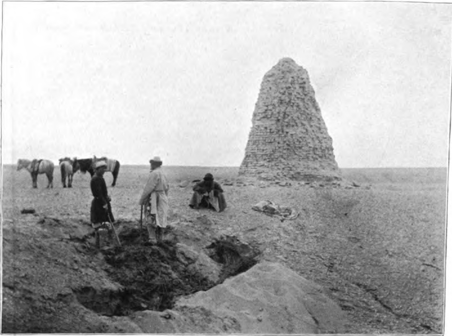
153. RUIN OF ANCIENT WATCH-TOWER T. III., NEAR WESTERN END OF TUN-HUANG LIMES. The spot where the first discovery of an early Chinese record on wood was made is marked by the two men in foreground.
